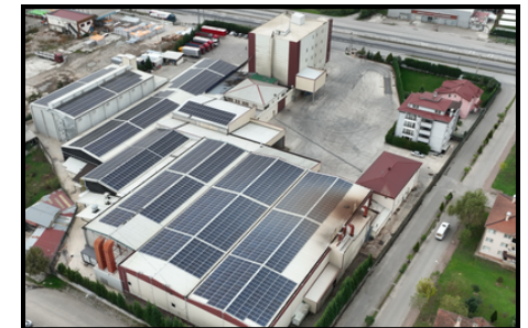
Durak Hazelnuts- Sakarya/ Hendek Cracking Plant
