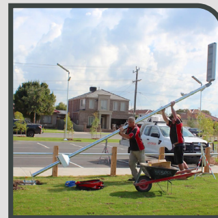
3. Raise into place
