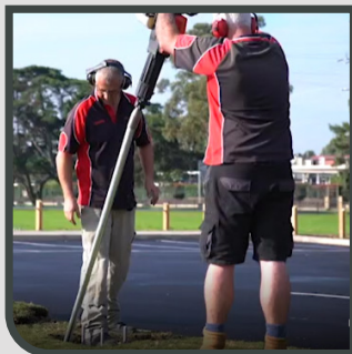
1. Concrete-less footings
