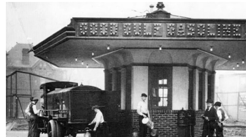
First service station opened by Standard Oil in Seattle in 1907
