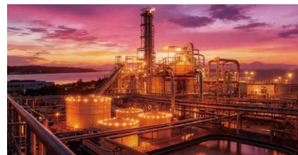
Chemical Processing Facilities: Delivering reliable emergency lighting in hazardous chemical environments to support safe movement and quick response when normal power fails.
