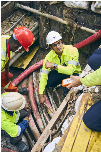
Work below ground
