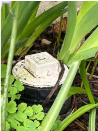
Image 1.11.1 Drain clean out located along the south wall of the house.
