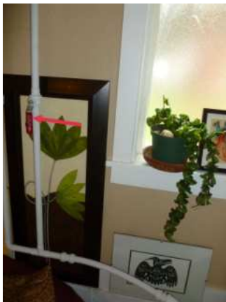
Image 5.5.1 Shut off ball valve
