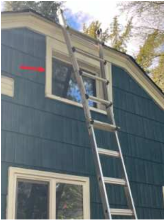
Image 7.3.1 Attic access located outside on east facing wall.
