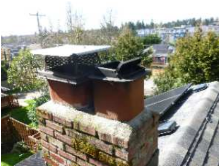
Image 2.5.1 Chimney cap present
