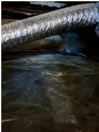
Image 8.3.1 Poly vapor barrier in crawl space
