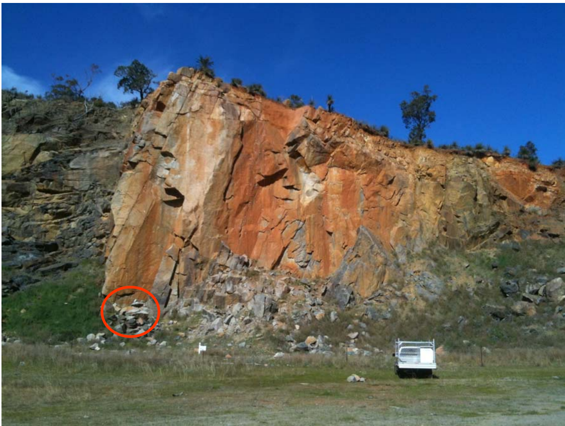
Top: Skywalker Wall on 15th July 2012. Red circle indicates the location of the block still attached. Bottom: Skywalker Wall on 29th July 2012. Red circle indicates the fresh rubble from the rock fall.
