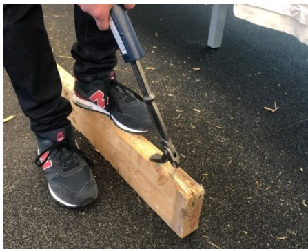
Removing fasteners
