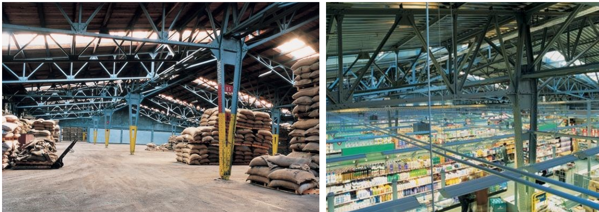
Figure 14. Original steel structure of Argentinian Warehouse (left) and reused steel structure in Brazilian Shopping Center (right), Amsterdam [99]
