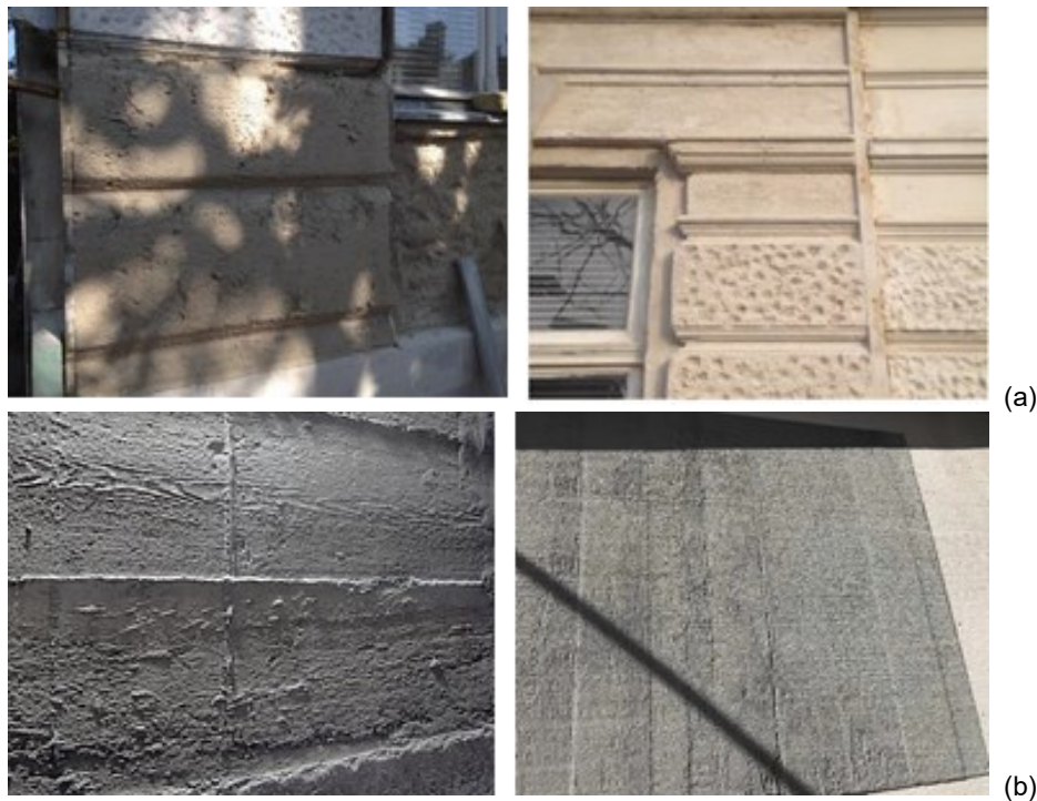
Figure 2. Visual comparison of façades in case of original materials and aerogel plaster application: (a) Renaissance building façade; (b) natural concrete façade
