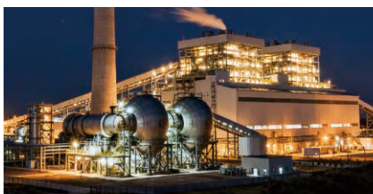
Power Plants: Providing robust lighting around high-risk equipment to support safe inspection and maintenance in demanding conditions.
