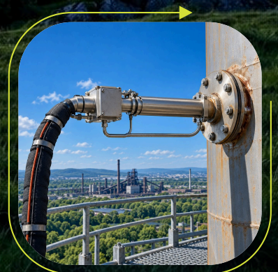
STACK EMISSION MONITORING
