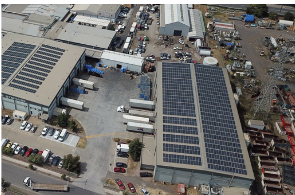
Solar PV - Ariel View 1
