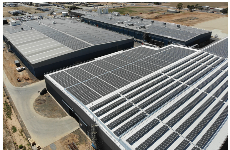
Solar PV - Ariel View
