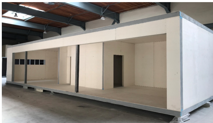
FRP structural frame assembled with insulated wall and roof panels, forming the main modular shell of the house.
