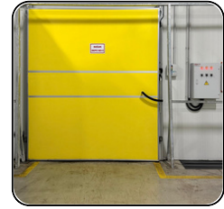
Cold Storage Room No. 5
