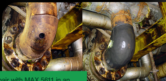
Oil leak repair with MAX 5611 in an offshore pipe bend.
