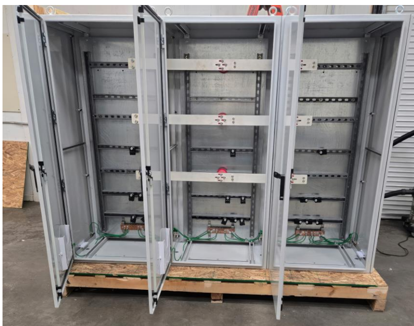
Figure 4 - Final Checks of Manufactured Splice Cabinet Before Shipment to Site
