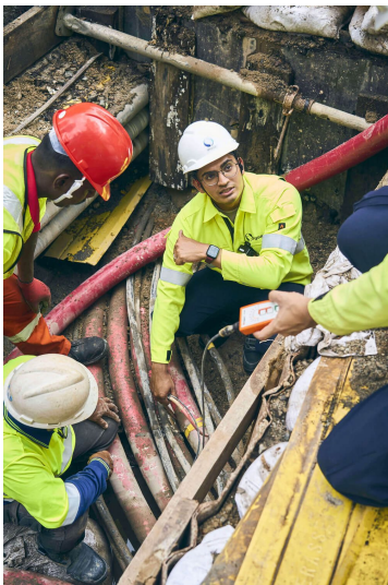
Work below ground
