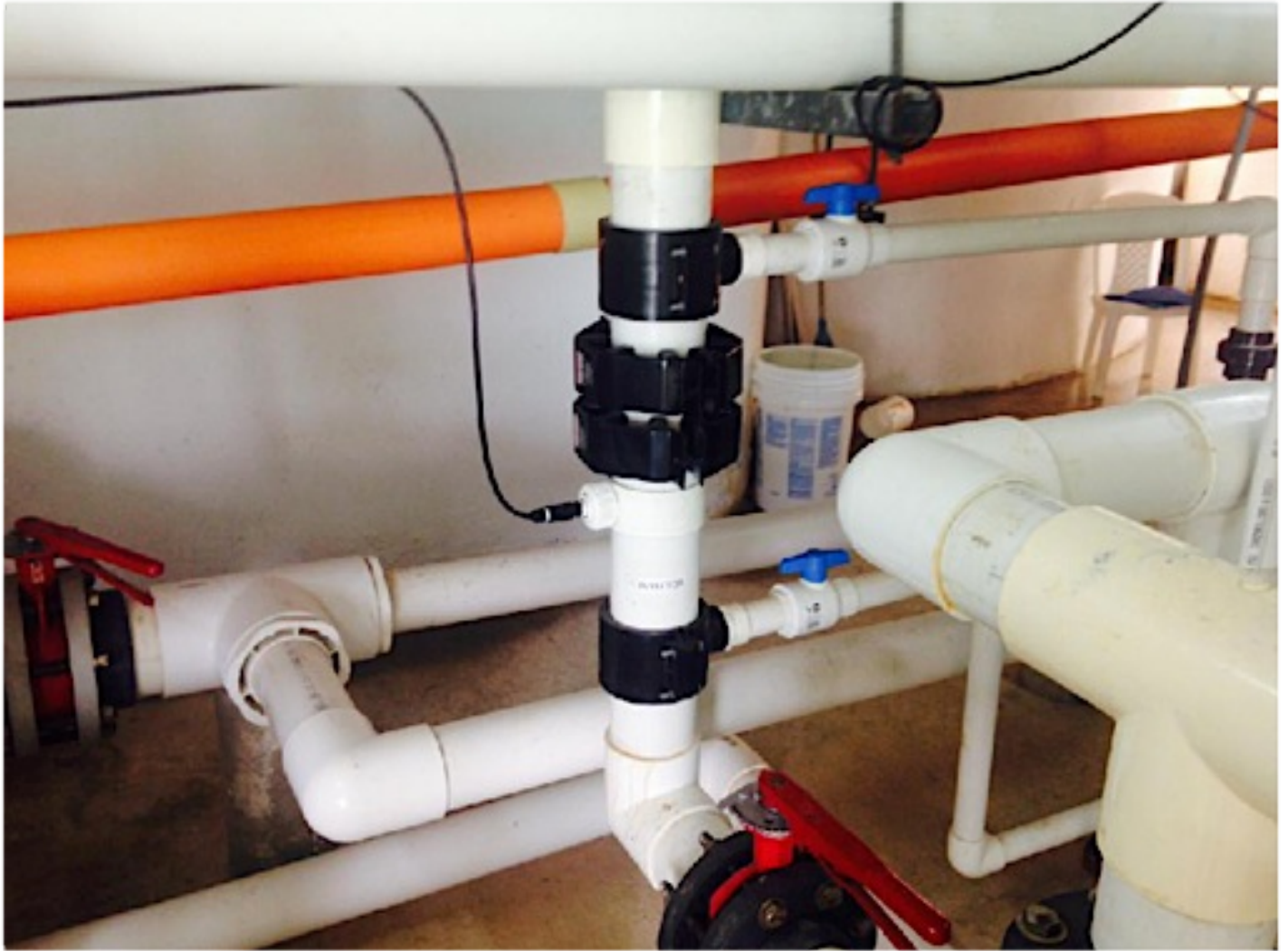
Magnetizer installation on 4" PVC pipe.
