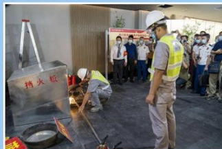
Hot Work Monitoring
