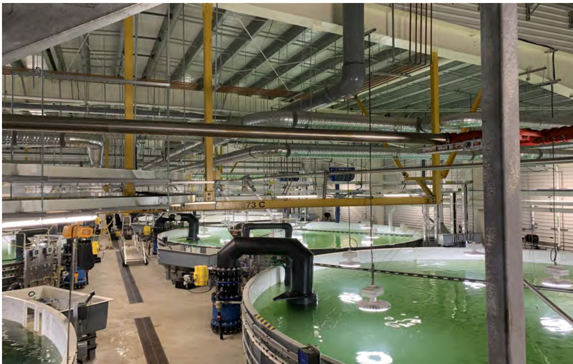
Figure 23. Innovation in resource efficiency: view of advanced recirculating aquaculture system for farm-raised salmon. This technology reduces freshwater use by 90%.
