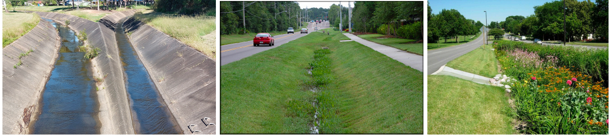
Figure B8. Examples of concrete channels, vegetated swales, and bioswales from left to right. (Penrith City Council, Brock University, Chapel Valley Landscape Company).
