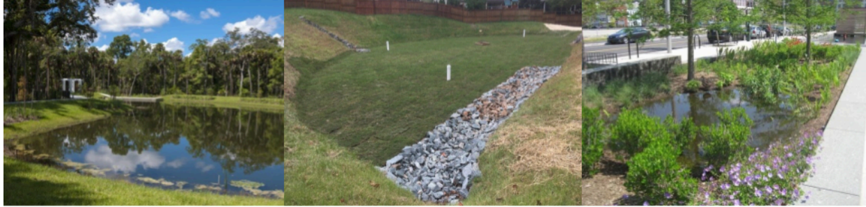
Figure B3. Examples of wet detention ponds, bioretention basins, and rain gardens. (Professional Waterfront Cleanup, Dragonfly Pond Works, Pratt.)
