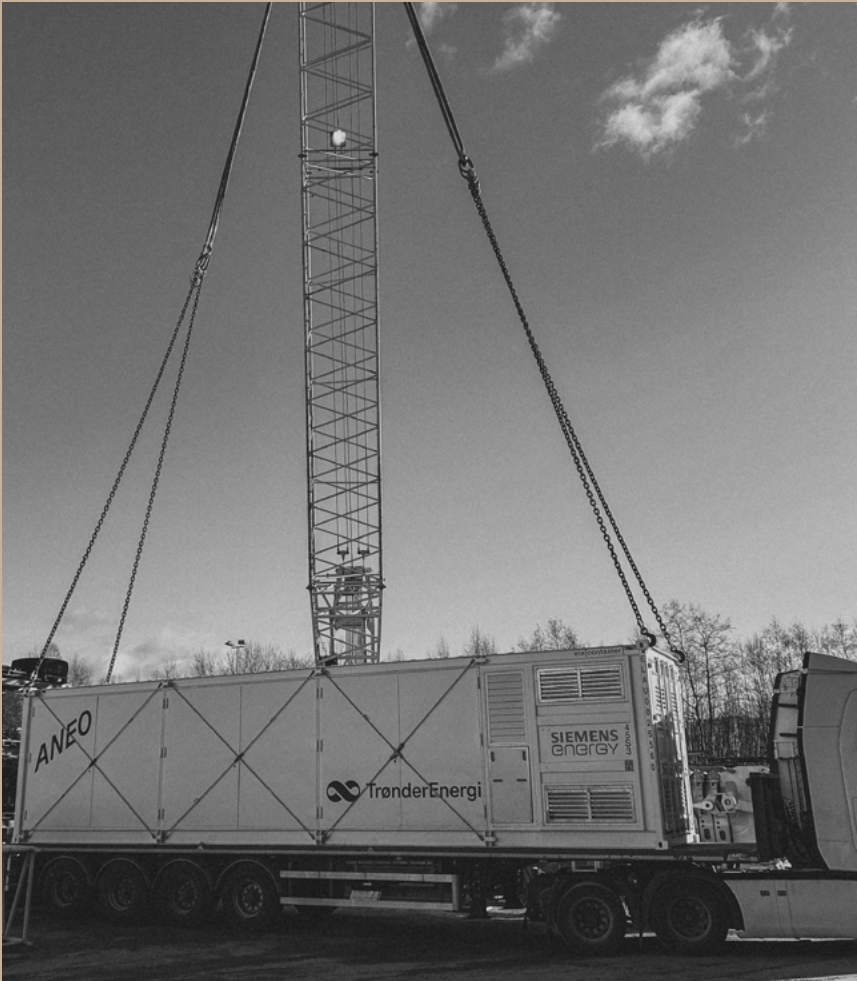
INSTALLATION OF THE BATTERY, DELIVERED BY SIEMENS ENERGY.
