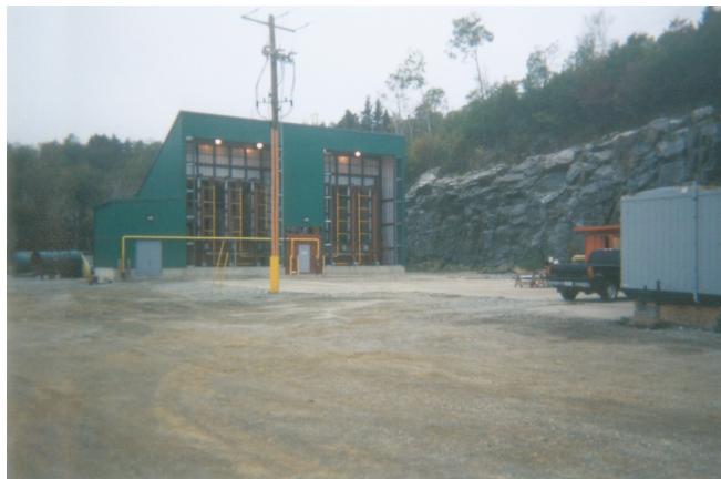
Figure 1 – Typical Mine Heater House
