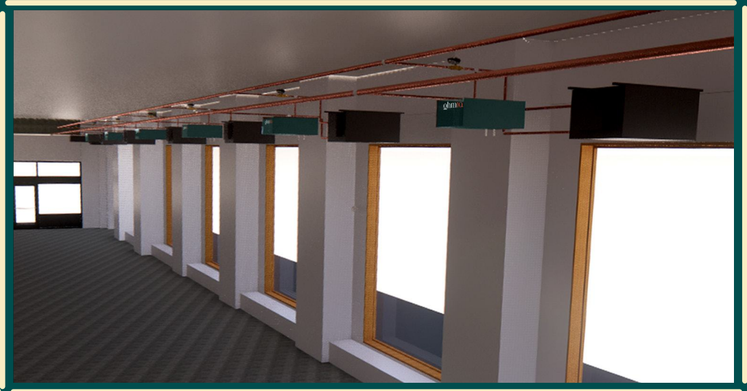
A TYPICAL FLOOR PLATE WITH A THERMIQ UNIT INTEGRATED WITH THE TERMINAL END UNIT FOR HYDRONIC DISTRIBUTION
