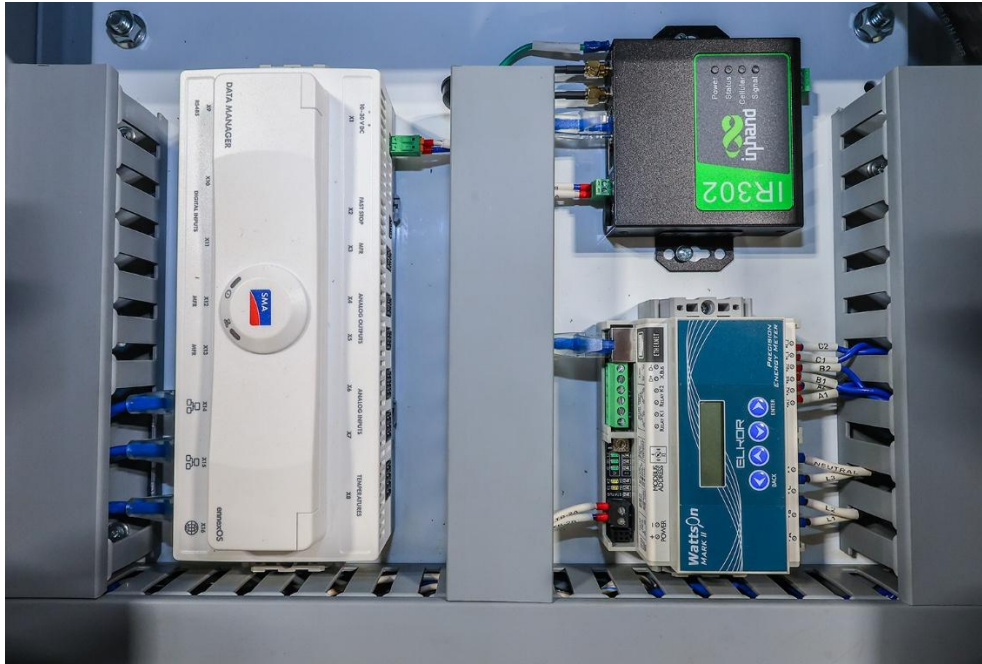
Figure 4 – Focus on Solar Command and Control Platform, Revenue-Grade Data Acquisition, and Cellular Router
