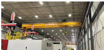
Industrial Plants & Manufacturing Workshops: High-bay environments resistant to dust, vibration, and temperature variations.
