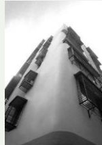
Rahul Apartments Dadar
