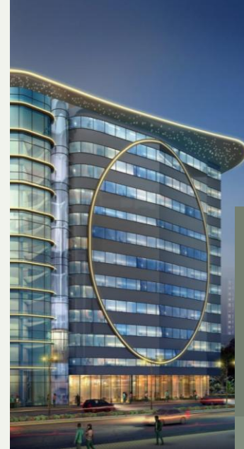
SARASWAT BANK DADAR WEST
