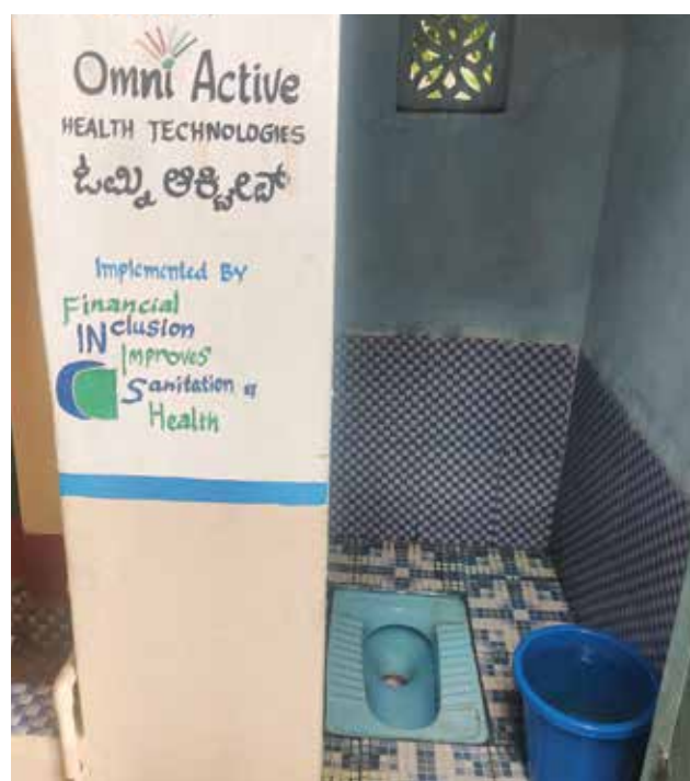
Anganwadi Kendra 1 Toilet in Berambadi
