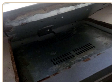
Rust on cooktop cut-out
