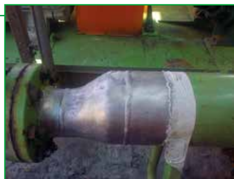
Reduction area with abrasive blasting
