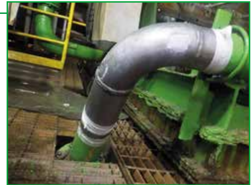
90° bend with abrasive blasting
