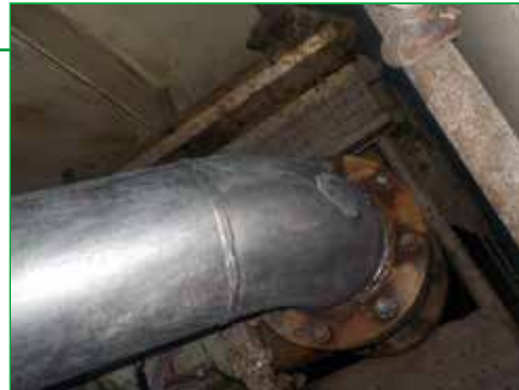
Abrasive blasting cleaning the surface
