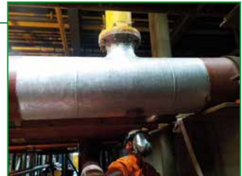
Reduction area with abrasive blasting
