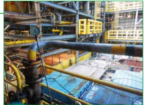
Abrasive blasting leveling the surface
