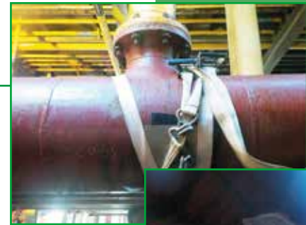
temporary structure reinforcement in the Tee...
