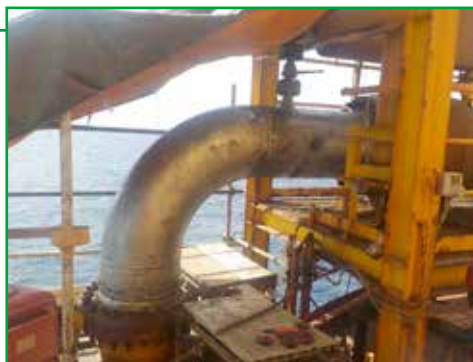
90° bend with abrasive blasting
