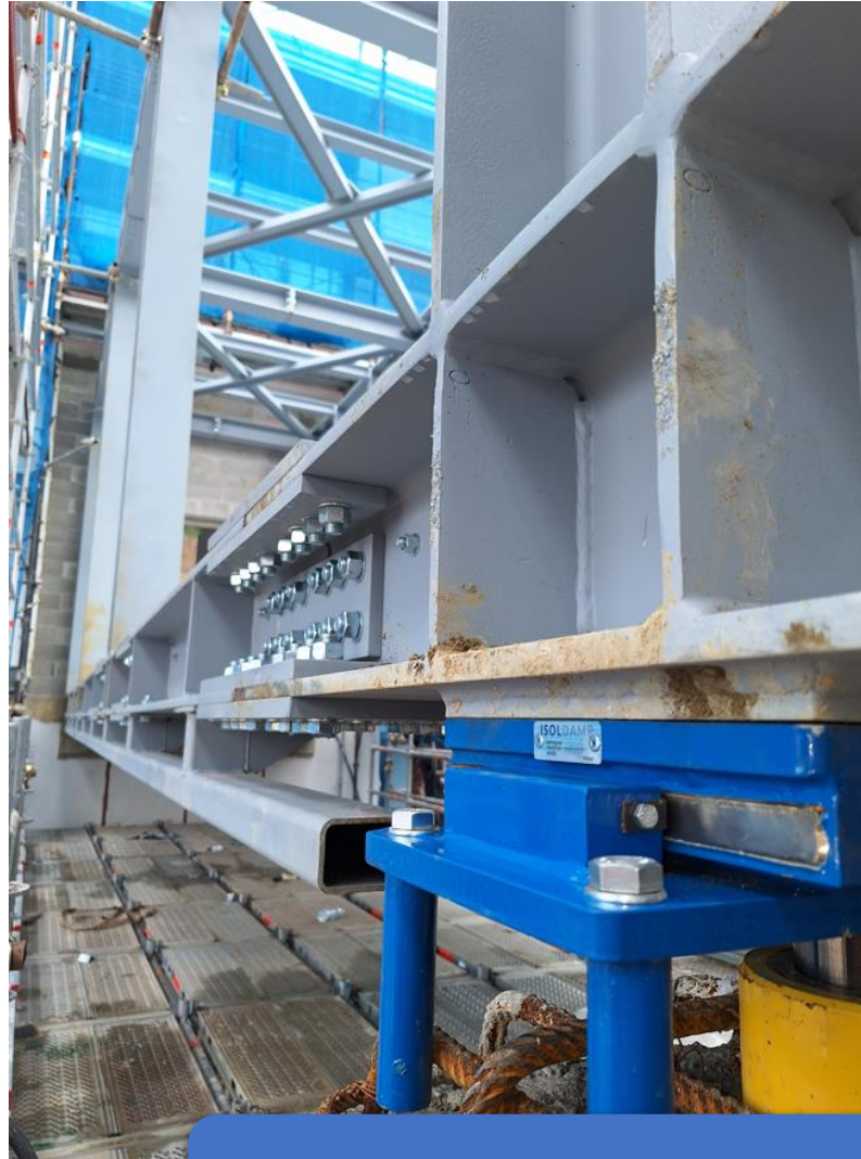
Humanitas PROTON Passengers bridge
