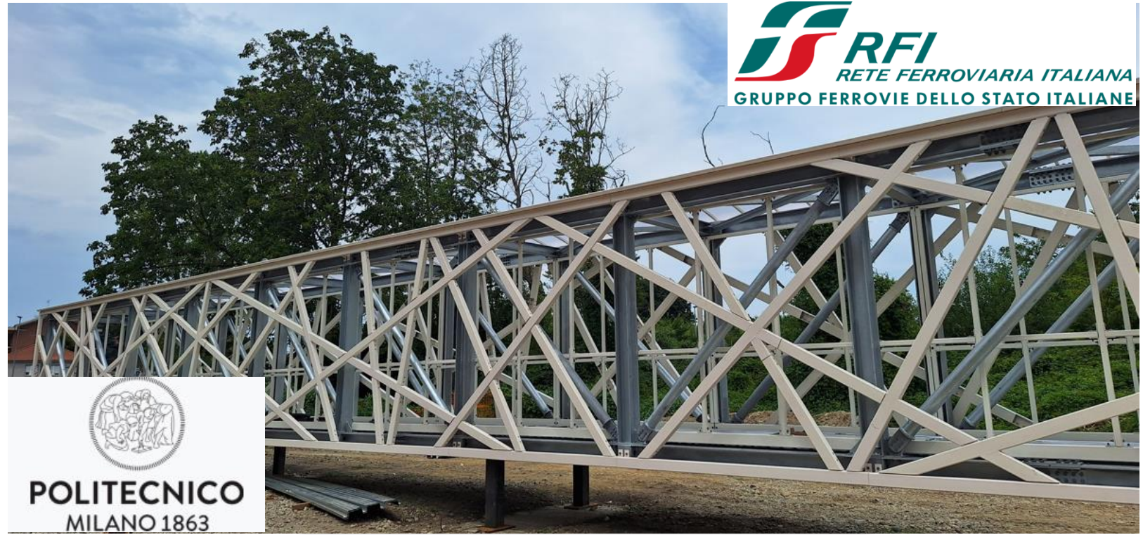
Passenger Bridge over Chivasso Railway station
