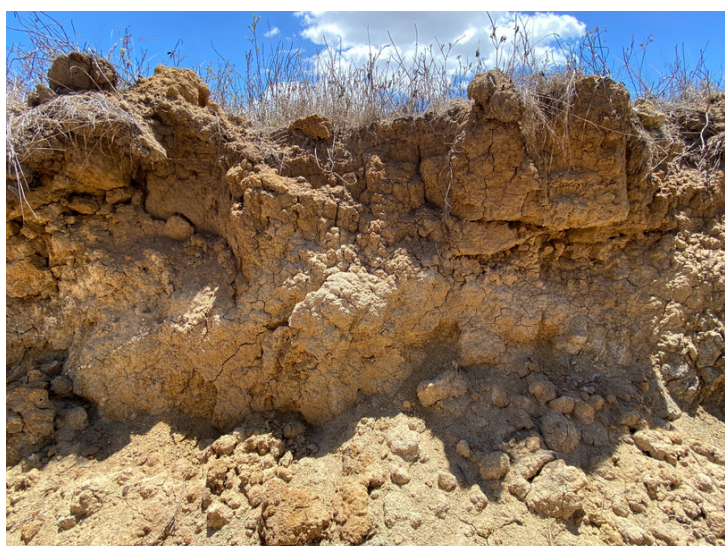
Figure 4. (Left) Slumping of the swale walls reflect the poor soil structure associated with sodicity.
