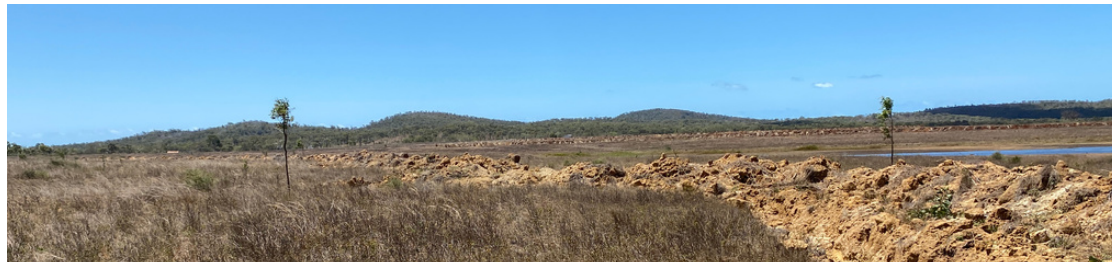
Figure 3. (Right) A newly constructed narrower and deeper swale.
