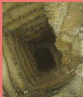
Figure 1.6 Cooling tower pack boroscope pictures
