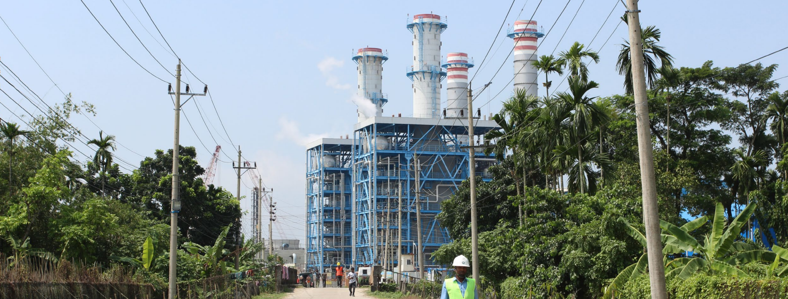
Bhola-2 220MW Combined Cycle Power Plant in Bangladesh was supported by the AIIB, MIGA, and other public financiers. Photo by Petra Kjell Wright, Recourse.
