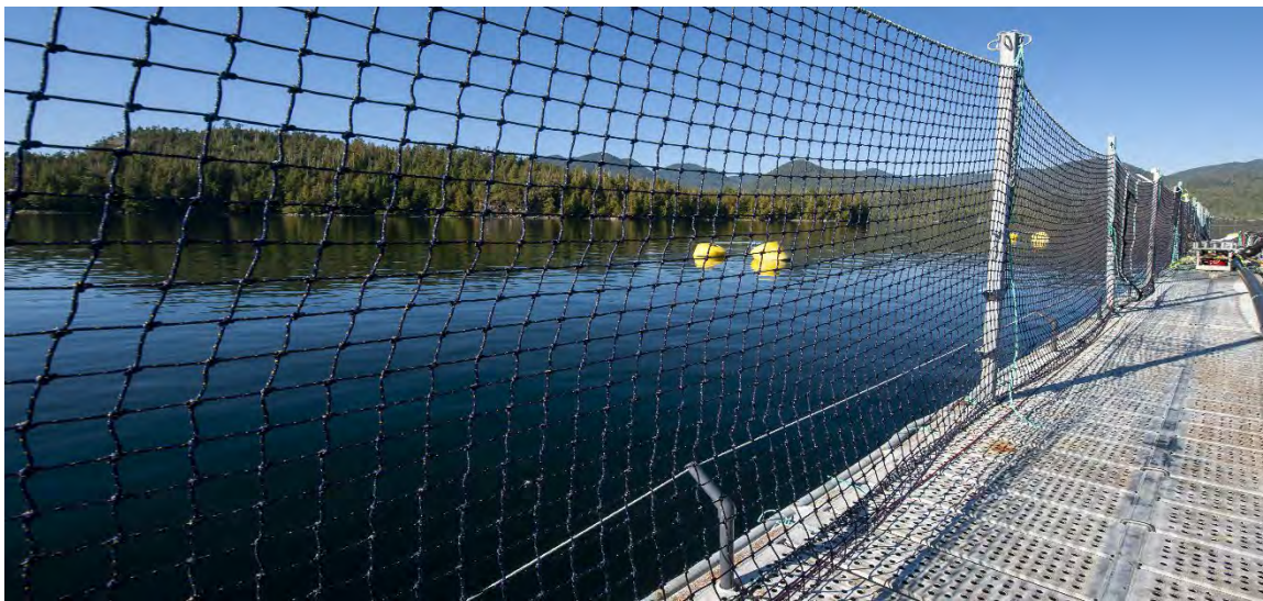
Figure 12. Electric line along outside of perimeter fencing.
