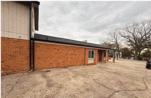
SIDE FACADE FACING THE STREET
