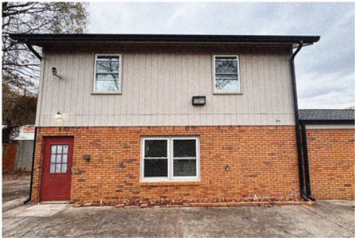
SIDE FACADE WITH THE TWO-FLOOR VOLUME
