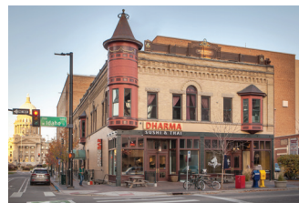
Adelmann Building Boise, Idaho
