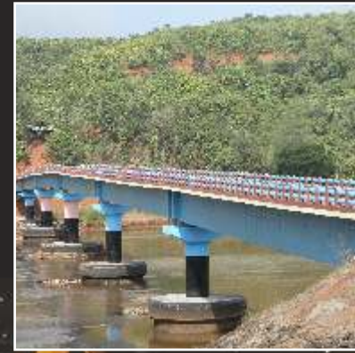
CHAMARSIL RIVER BRIDGE
