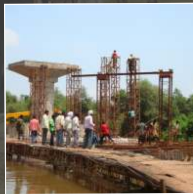
CUMBURJA CREEK BRIDGE GOA
