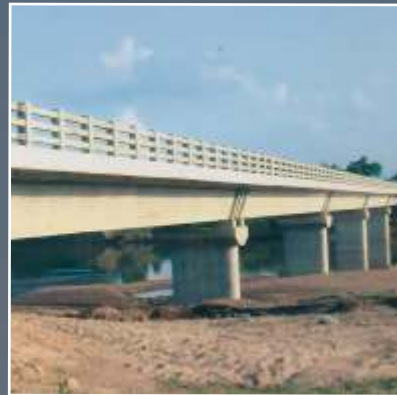
DEO-II (PIPERTOLA) RIVER BRIDGE
