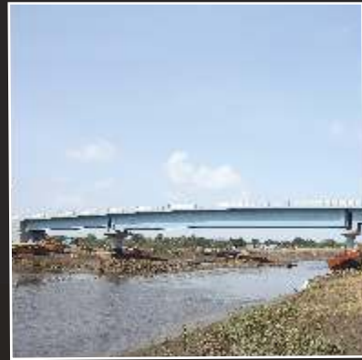
DOODH CREEK BRIDGE
