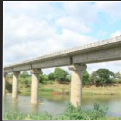
KRISHNA RIVER BRIDGE
