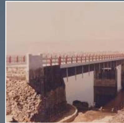
TALOJA CREEK BRIDGE
