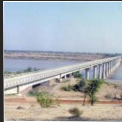
NARMADA RIVER BRIDGE
