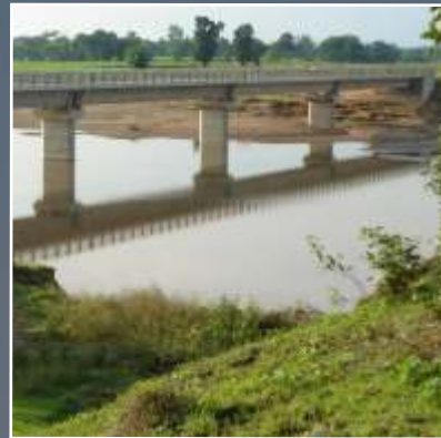
DEO-I (MURRI) RIVER BRIDGE
