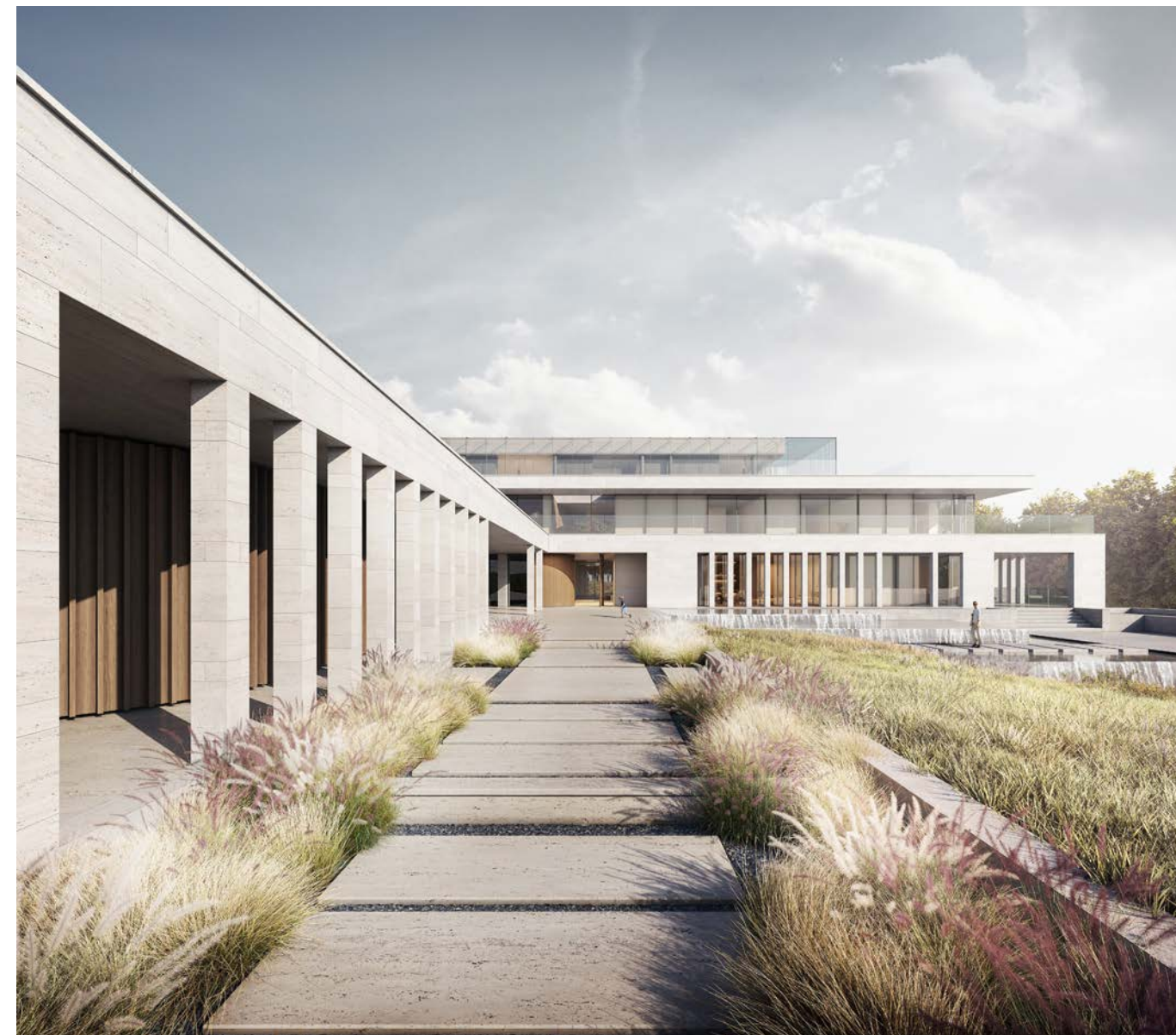
B house, Preston (under construction)
