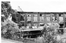
Abandoned Industrial Buildings
