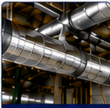
HVAC DUCT INSULATION
