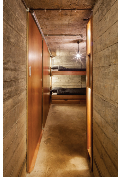
War Bunker Refurbishment-B-ILD
