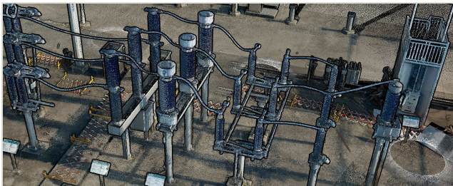
SUBSTATION DIGITAL TWIN, PHOTOREAL POINT CLOUD
