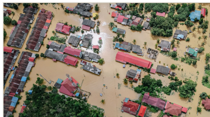
INUNDATION EXTENT MAPPED BUILDING BY BUILDING
