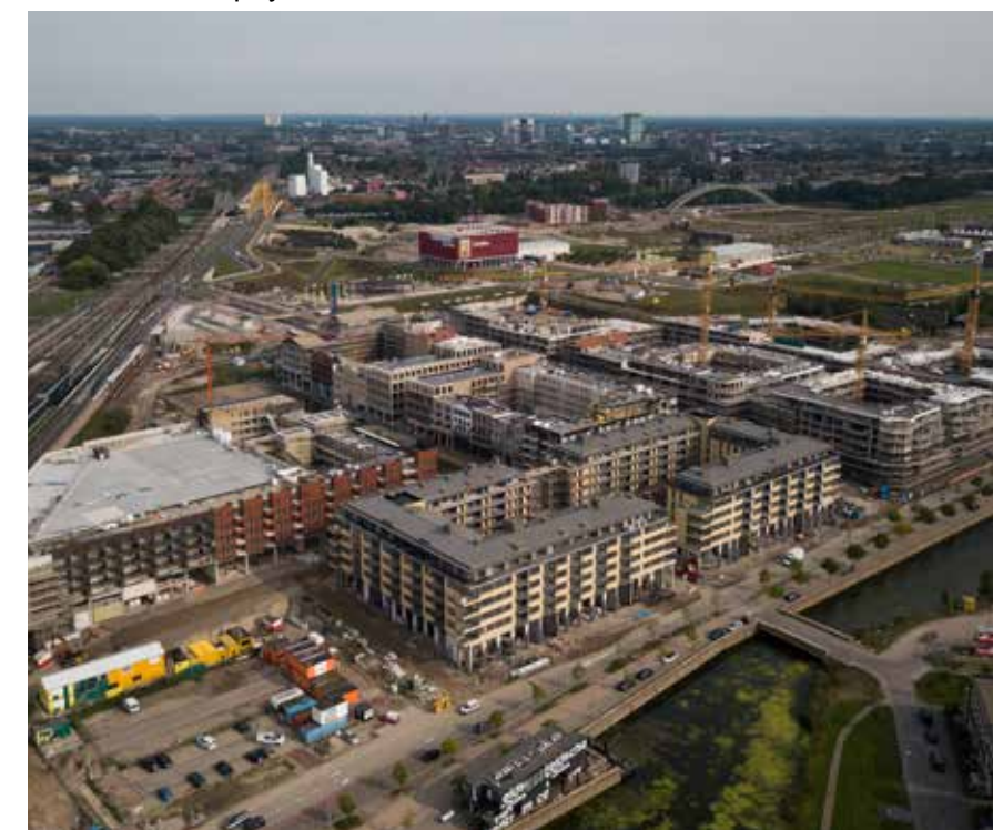
An overview of the project
