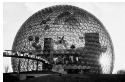
A geodesic dome designed by Buckminster Fuller as the U.S. pavilion at Expo 67 Montreal, 1967. © Estate of R. Buckminster Fuller.
