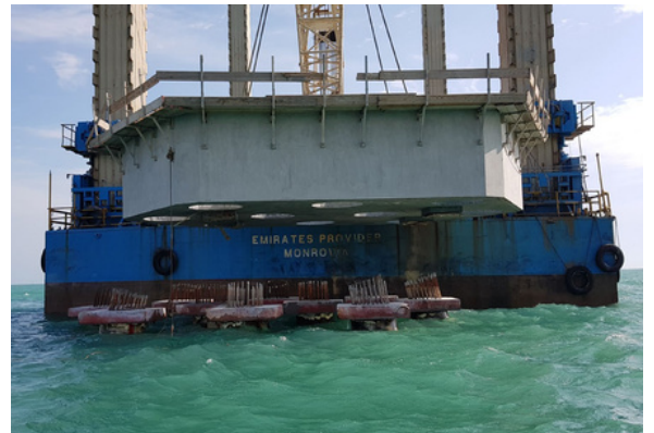
Construction of Dolphins for Cruise Terminal at Old Doha Port
