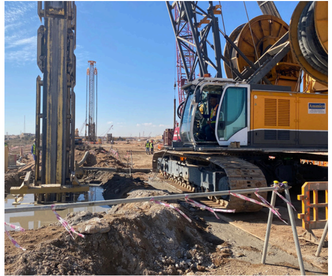
Cut-off Wall at The Line – NEOM, KSA
