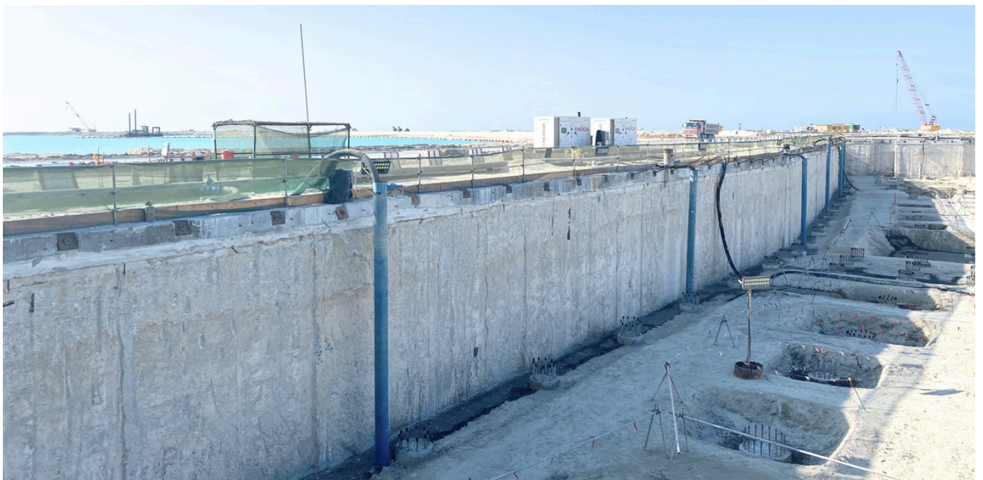
CSM Wall Face after Excavation, Laheq Island – Red Sea, KSA
