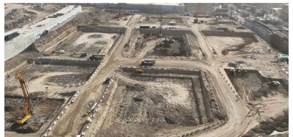
Rigid Inclusions at Superblock 5 – Rua Al Madinah, KSA
