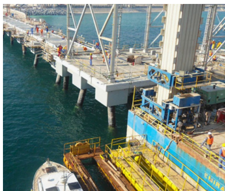
Construction of Jetty – Gas Sweetening Facility - QP - Mesaieed, Qatar
