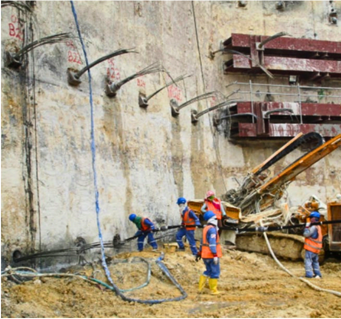
Installation of Ground Anchors – Doha Metro – Msheireb Station
