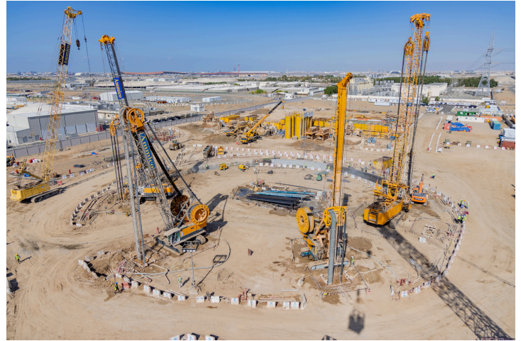
100m Deep Diaphragm Wall for North Jeddah Pump Station
