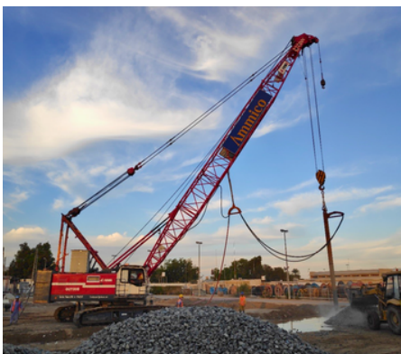
Stone Columns at Desalination Plant – Kalba, Sharjah, UAE
