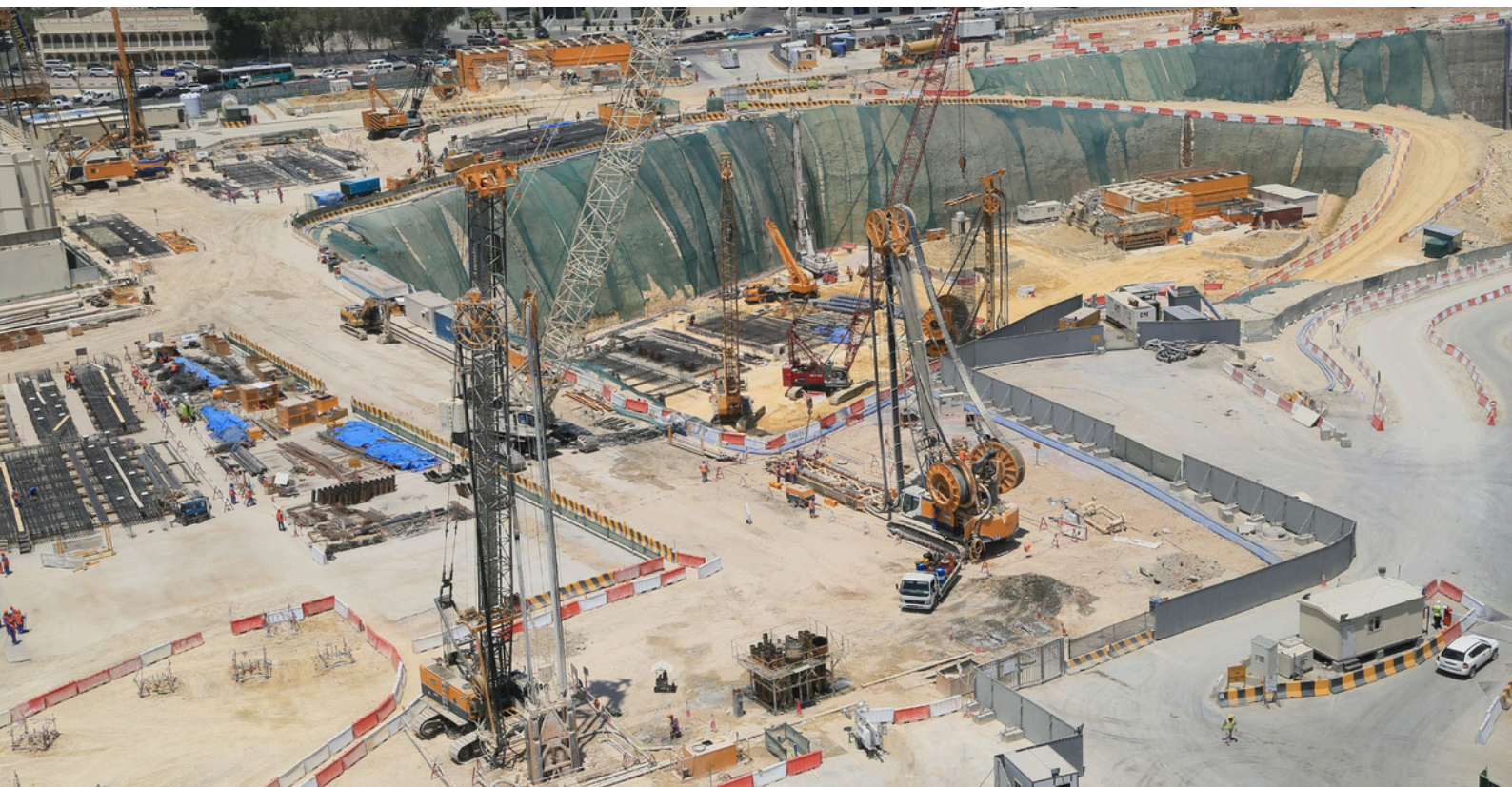
Diaphragm Wall, Excavation & Anchoring Works – Doha Metro – Musheireb Station
