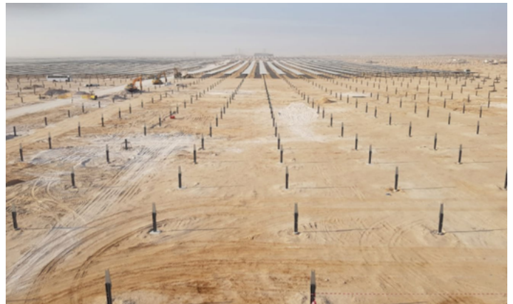
Installation of Micropiles and Posts Solar Plant at Al-Kharsaah, Qatar
