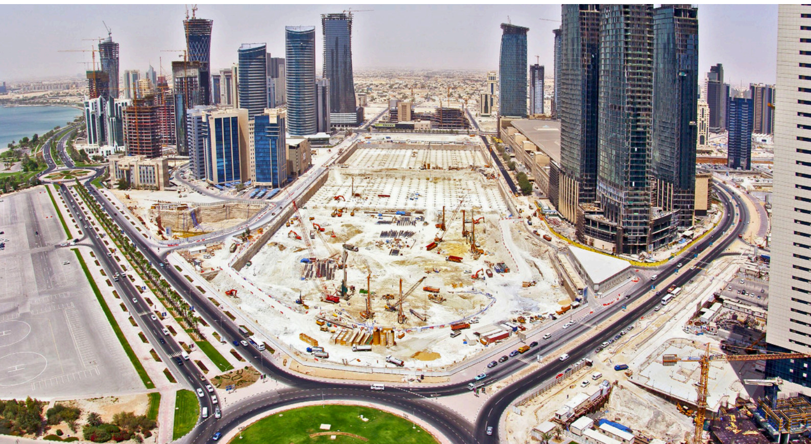
Enabling Works at Doha Convention Center and Tower
