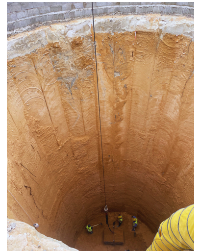
CSM Wall Installation Shafts for Storm Water Drainage Project – Qassim, KSA
