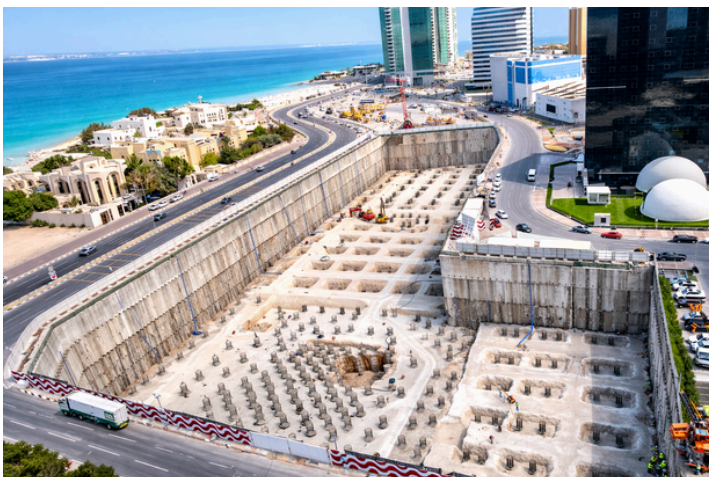
Enabling Works for Al-Quds Tower Project – Doha, Qatar
