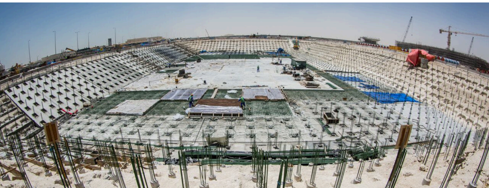
Installation of Micropiles – Water Mega Reservoir – Doha, Qatar
