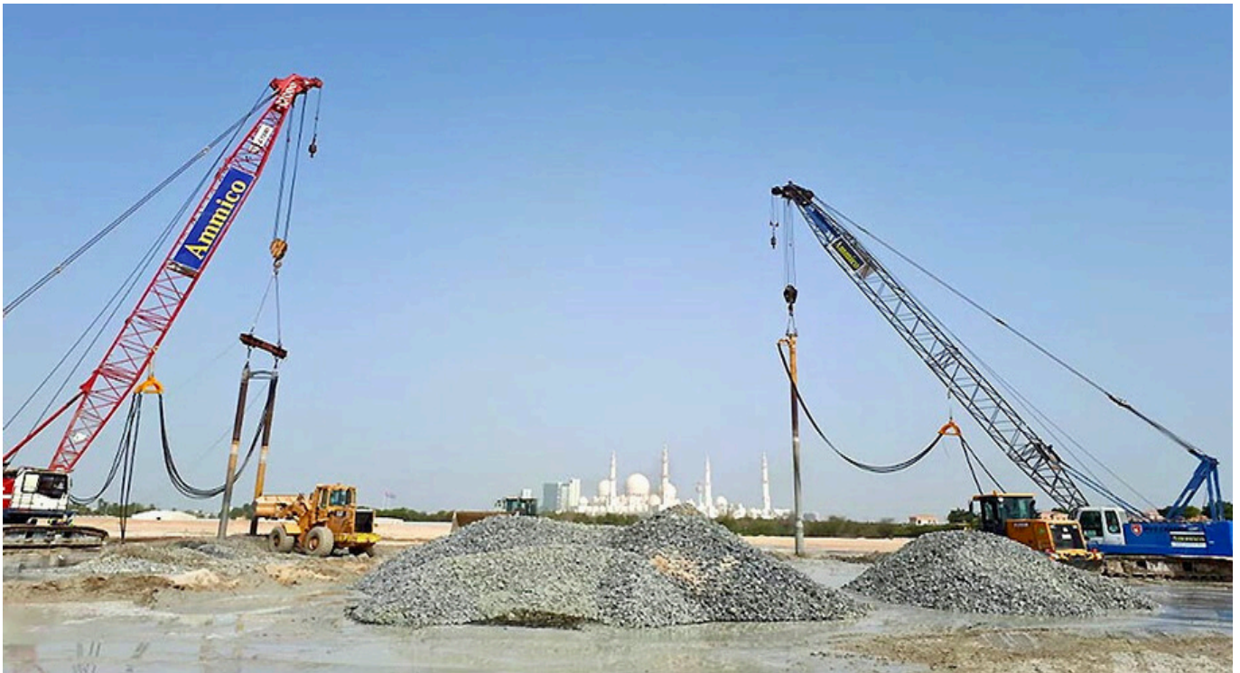
Installation of Stone Columns – Traditional Souq, Abu Dhabi
