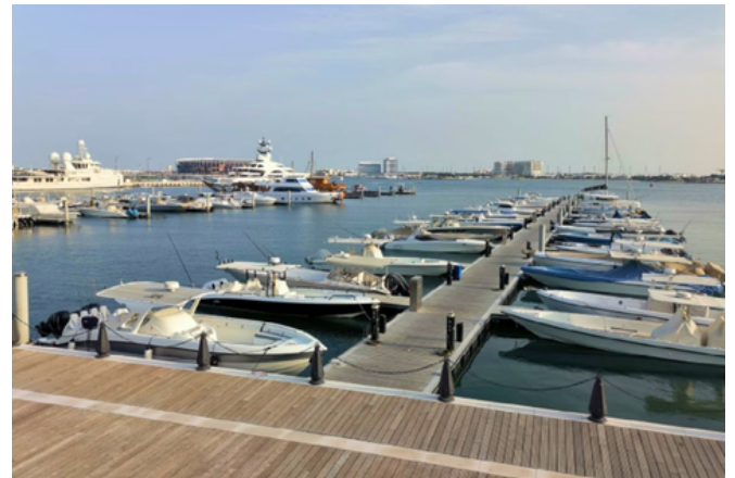
Construction of Marina at Old Doha Port
