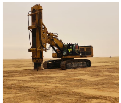
Rapid Impact Compaction (RIC) – Jafurah Gas Field – KSA
