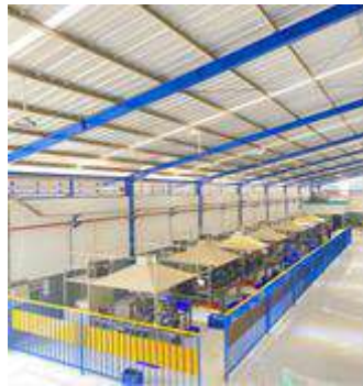
Line Robot Welding
