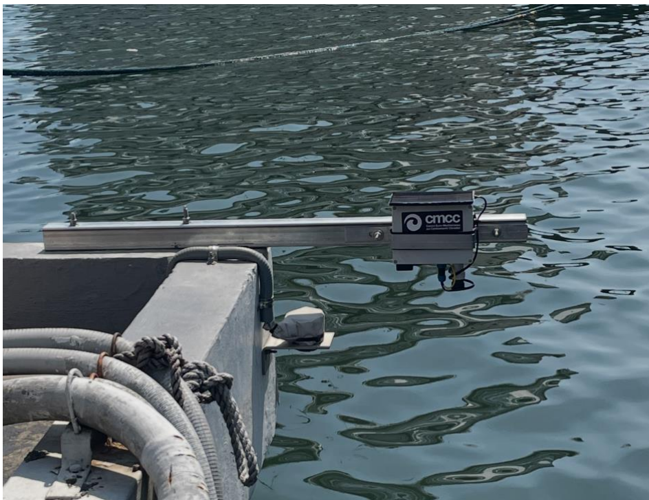
Figure 15. Installation of InterBox during training activities with master degree students
