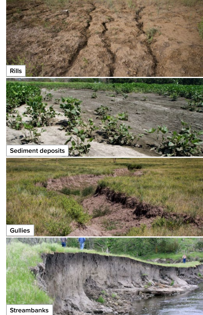
Figure 4.5d. Common erosion indicators
