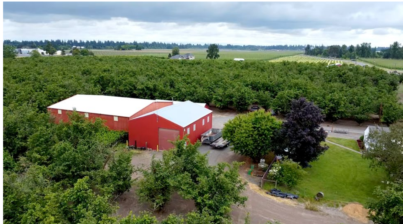
Right: Buildings and farm infrastructure should be evaluated for their opportunities and constraints.
