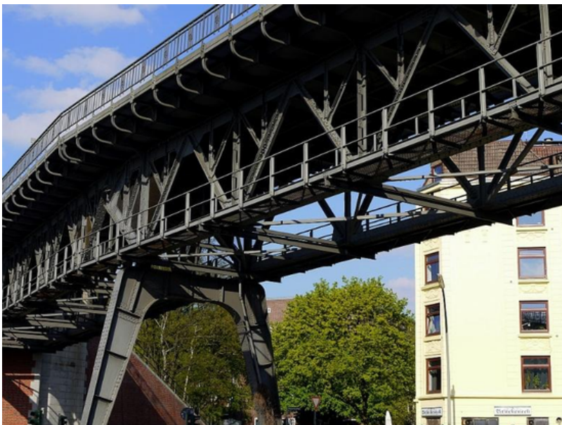
Viadukt in Hamburg-Barmbek (Ctsu / CC BY-SA 3.0)
